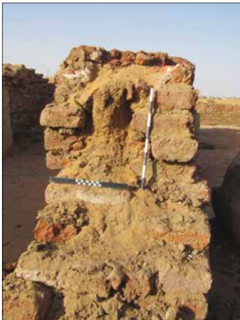
Plate 14. Foundation of the Phase III Church with fragment wooden pier still in situ (photo: Bogdan Żurawski).
