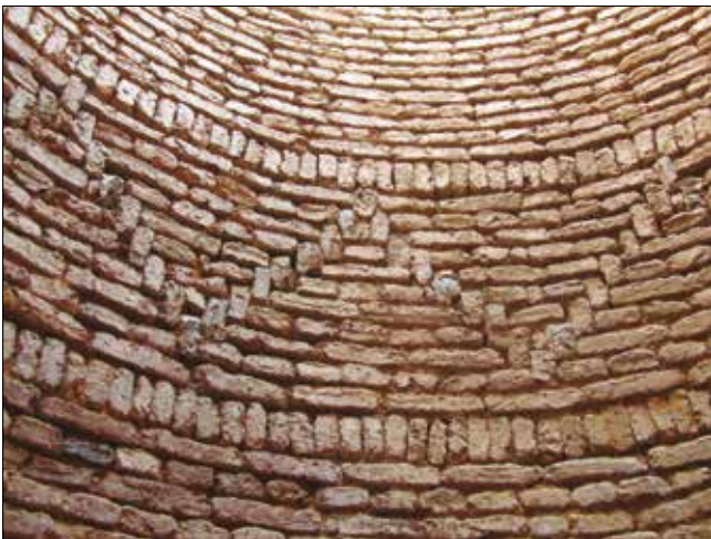
Plate 18. The zig-zag pattern made of overfired brick within the well at Selib 1 (photo: Bogdan Żurawski).
