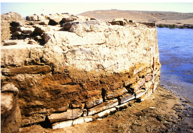
Figure 100. The exposed face of the round tower.
