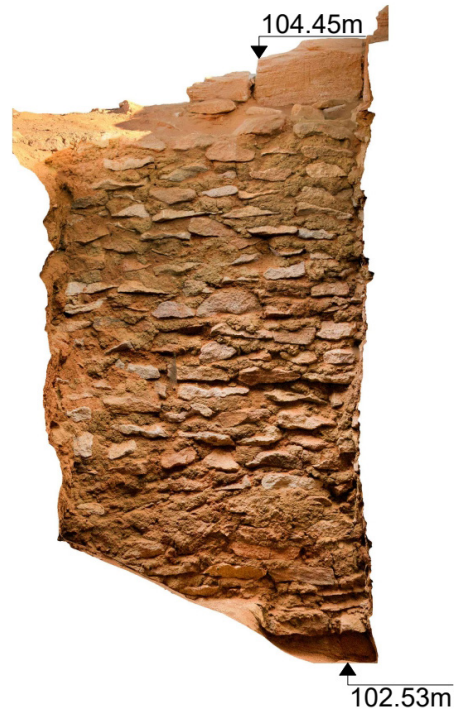
Figure 3. Section in the northeast corner of 1011 showing the foundation consisting of gravel at the bottom, rubble sandstone plates with tough clay between the layers, followed by roughly worked sandstone blocks, on top of which the first layer of the actual wall was placed. View from south to north. (© Naga Project).
