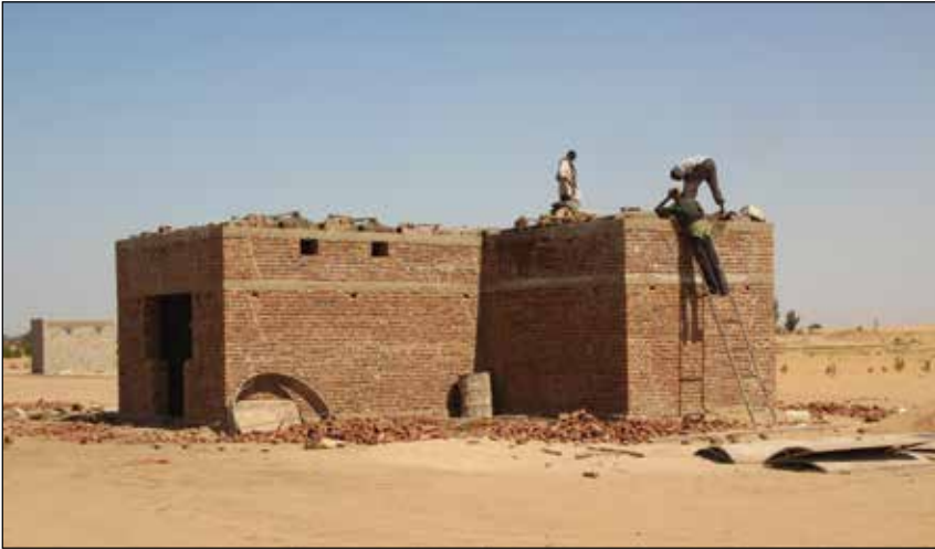
Plate 21. The Visitors' Centre; constructing the Libyan roof.
