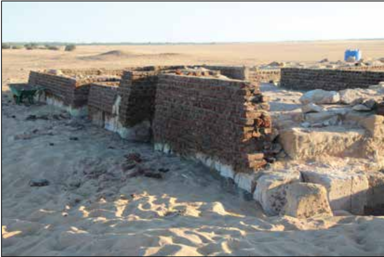
Plate 19. Temple T, modern walling under construction.
