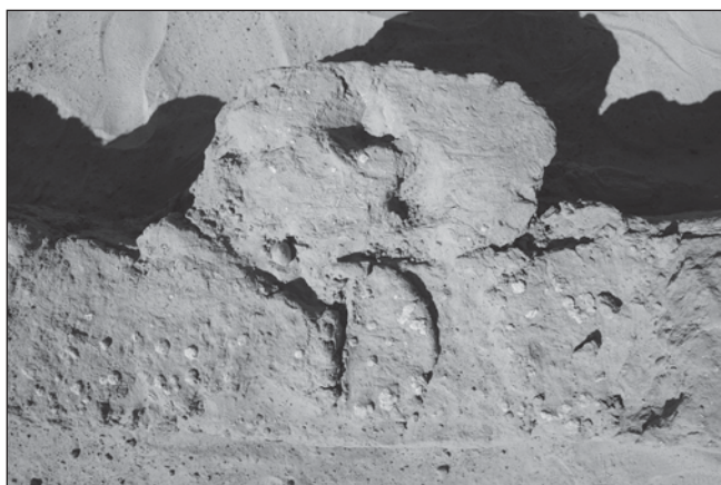
Plate 5. Detail of brickwork 2225, with a door-socket.
