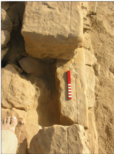
Plate 12. Setting out lines on the stepped courses of the small pyramid (Pyramid 1) in the Kushite cemetery at Kawa (photo D. A. Welsby).
