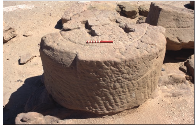
Plate 13. Dove-tailed cramps on a column drum from the portico of B700 at Jebel Barkal (photo D. A. Welsby).
