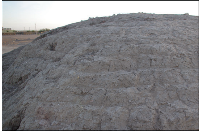
Plate 15. Close-up of structure with the stepped brick courses clearly visible.
