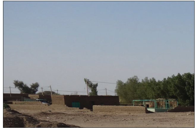
Plate 10. Construction and mortar preparation platform, facing southwest.
