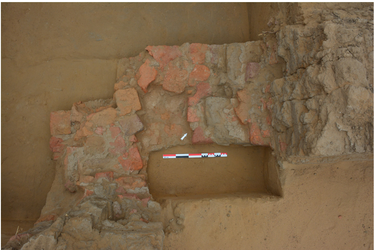
Figure 4. Corners F 006-F 010 (above) and F 010-F 013 (below) showing broken red bricks in the foundations of the new aisle (© SFDAS).
