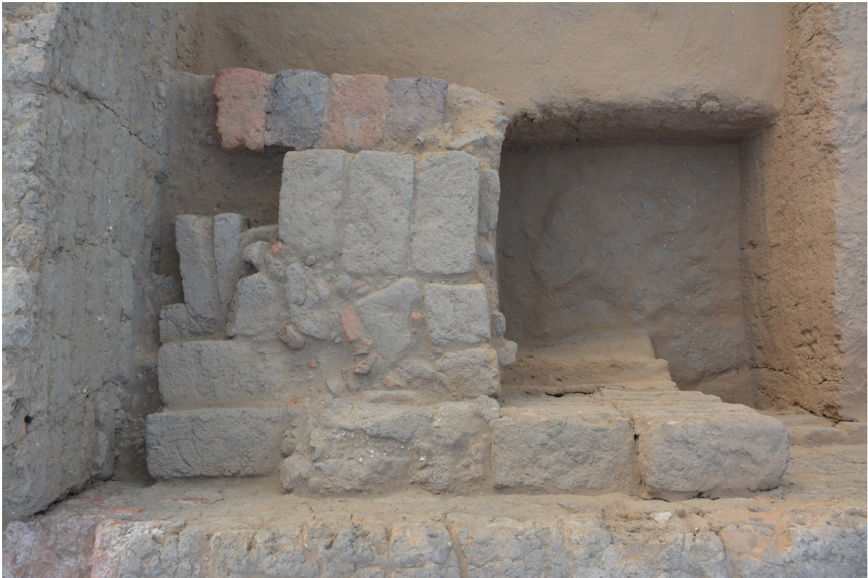
Figure 7. Staircase F 087, view from above (© SFDAS).
