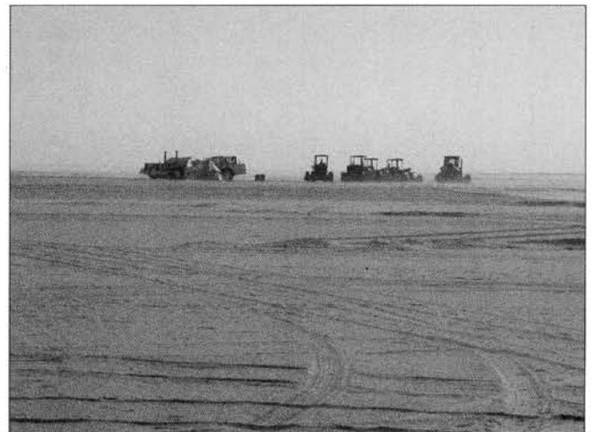
Plate 1. Bulldozers at work in the scheme.
