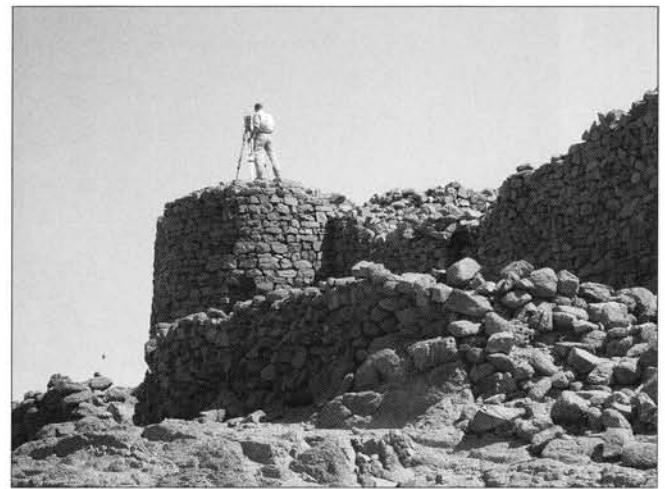
Plate 11. Survey work in progress on the north bastion of Haraz fortress.
