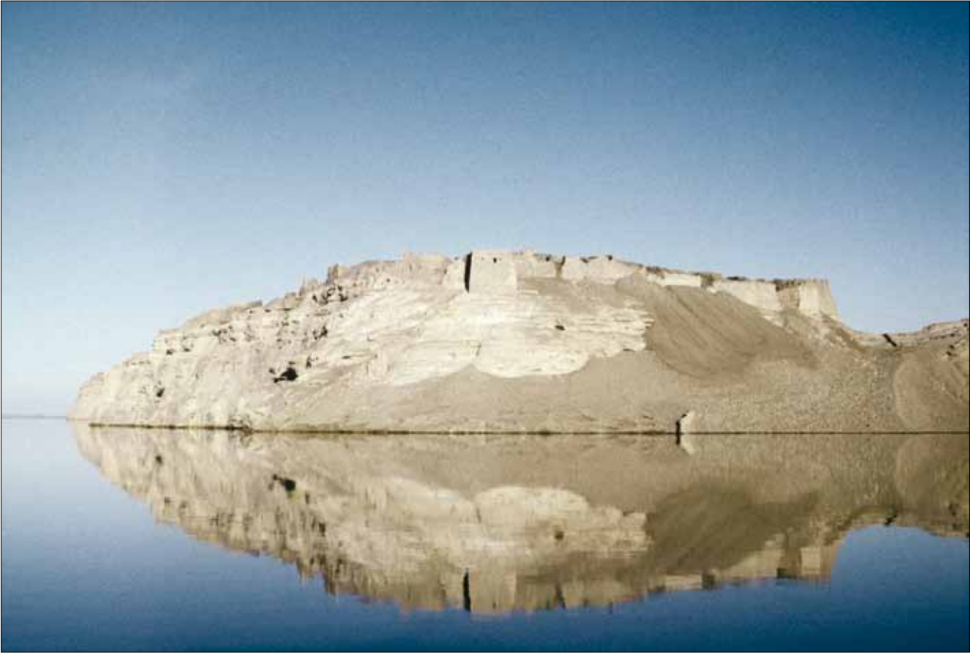
Plate 1. View of Qasr Ibrim as the waters of Lake Nasser were rising (1966).
