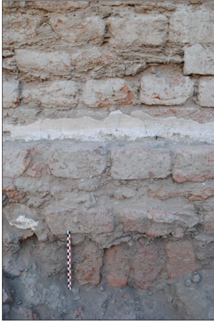
Plate 13. Red-brick foundation courses beneath temple wall.
