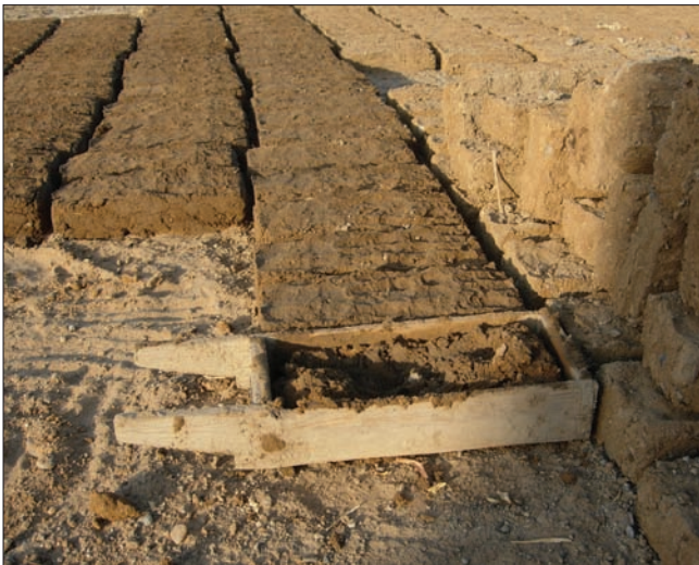
Plate 21. Modern wooden mould used for making mud bricks.
