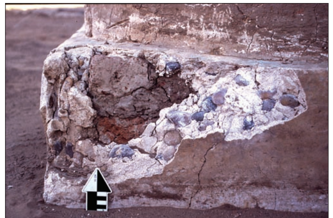
Plate 6. Cement consisting of lime and rounded pebbles on a column base in the first court.
