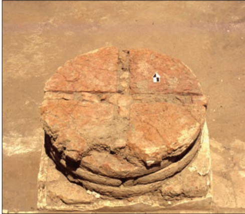
Plate 3. Column in the first court with galletting.
