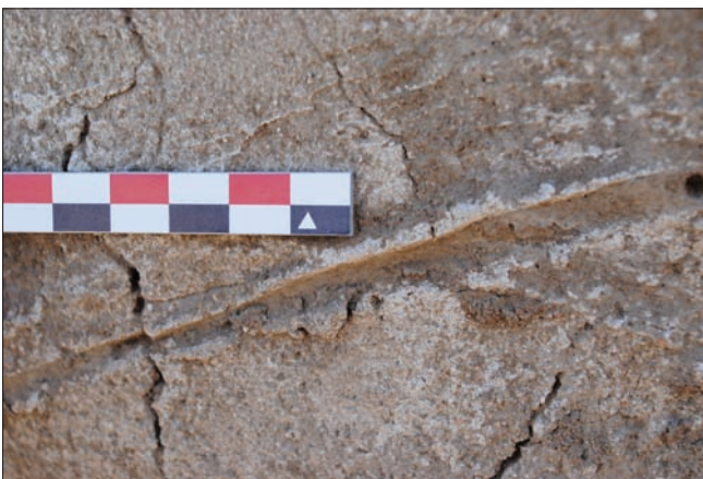
Plate 4. Lime-plaster scratch coat.
