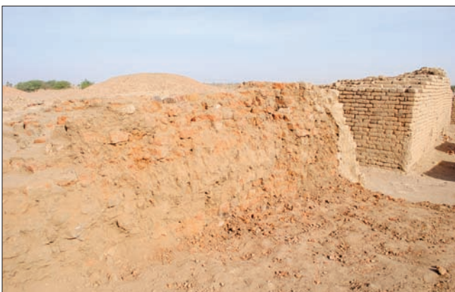
Plate 15. East face of the south pylon, with outer facing damaged or missing.
