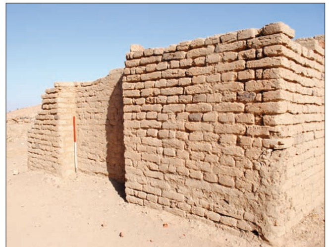
Plate 12. Brick work in the north pylon (facing north west).
