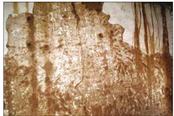
Plate 10. Part of an old wall inside Khalwat El-Sayid el-Hassan.
